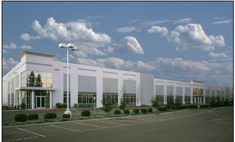
Herakles Data's 52,500-sq ft co-location data center in Sacramento, California.
