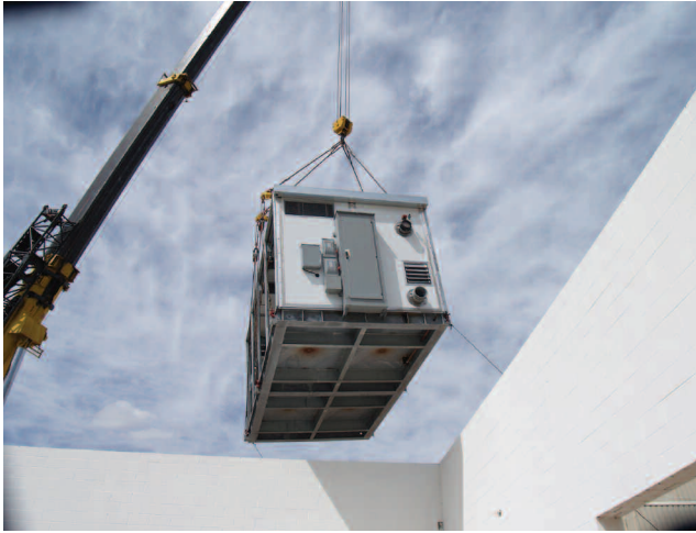
The McQuay Modular Central Plant arrives at the jobsite as one pre-engineered and pre-assembled module, ready for final assembly and hook-ups.
