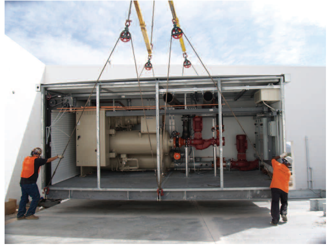
The McQuay Modular Central Plant arrives at the jobsite as one pre-engineered and pre-assembled module, ready for final assembly and hook-ups.
