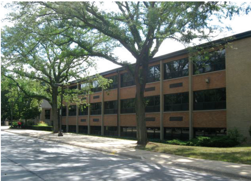
The two-story, 135,000-square foot Northbrook Junior High School was originally built in 1958 and now serves 650 students in grades six through eight. The renovation project included replacement of all heating and cooling system components.
