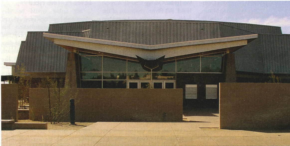
Since the commissioning of a modular central plant, Chaparral High School in Scottsdale, Ariz., has seen electrical savings of $800 a month over its old system, according to officials.
